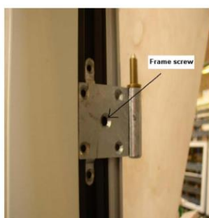
Figure 9. Mounting the doors
