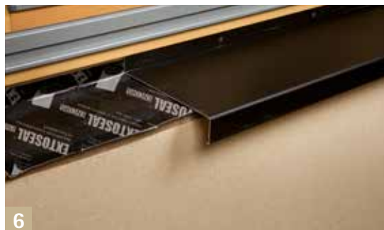
6 Install the window sill
