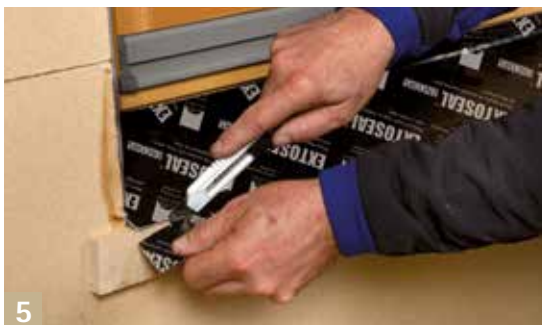
5 Cut off horizontal excess
