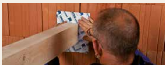
Beam penetration in masonry wall
