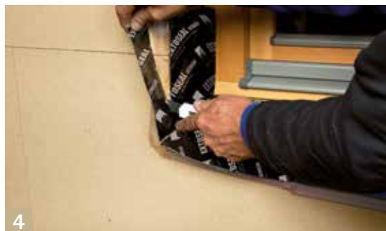
4 Cut off vertical excess
