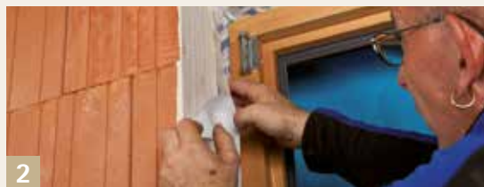
Stick to the soffit and rub on
