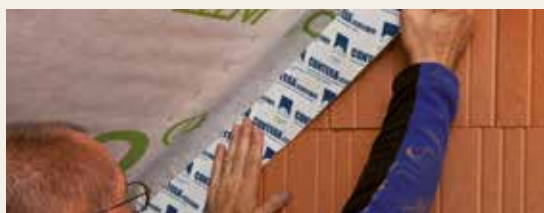
Masonry gable end wall, creating an airtight joint
