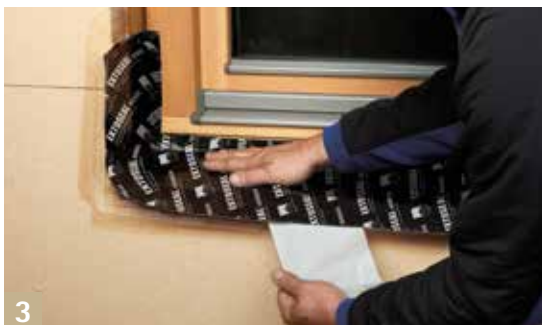
3 Tape in the soffit
